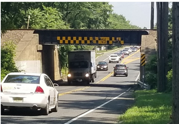
Photo 2 - NJ Transit Railroad Bridge (looking south)
