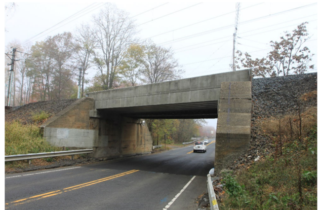
Photo 2 - 2022 Emergency Superstructure Repair (looking north)
