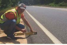
Example of the SafetyEdge<sup>sM</sup> after backfill material settles or erodes. Source: FHWA
