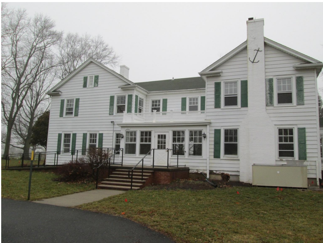
Hominy Hill Administration Building - January 2017
