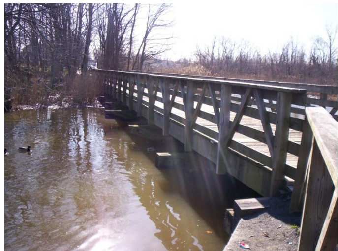
Bridge over Waackack Creek
