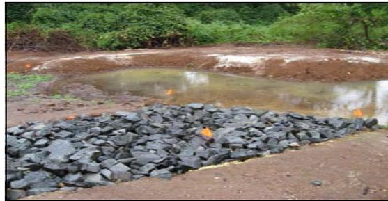
The garden after a 2 inch rainfall and before planting. Stormwater percolated into the ground within a few hours, leaving behind sediment & pollutants.
