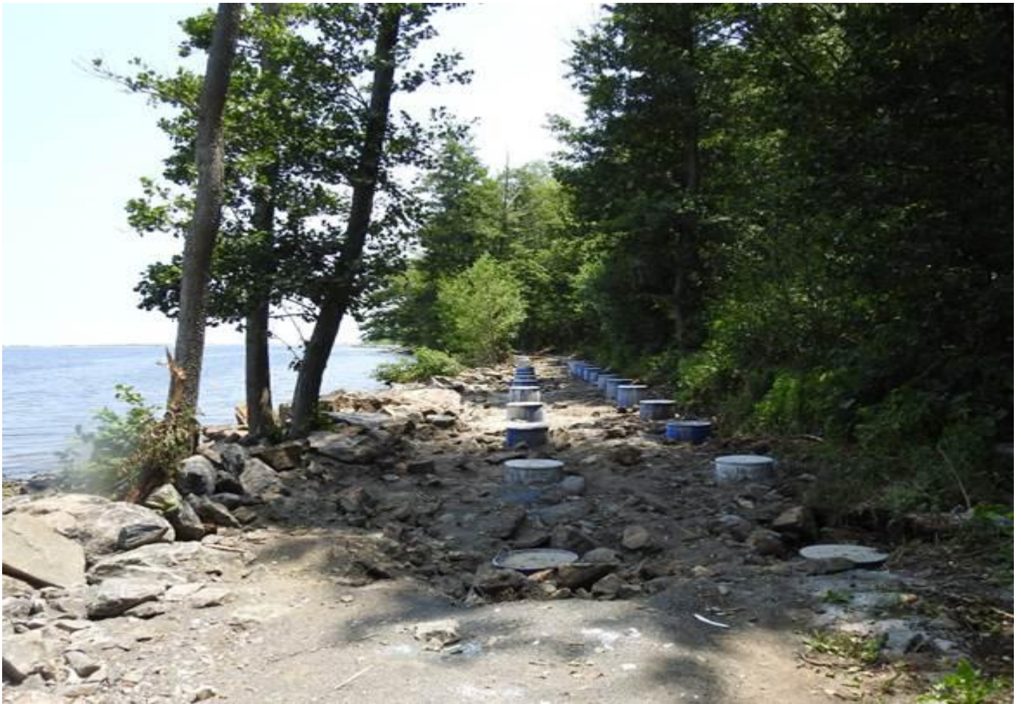
Piers for 1 of 5 Bridge/Boardwalks Installed
