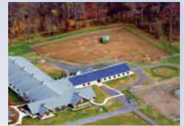
The Equestrian Facility at Sunnyside Recreation Area. Sunnyside was the first park site to install solar panels for energy, visible in this aerial photo.
