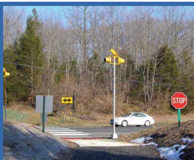
The UTT has an elaborate crossing over Route 539 involving plenty of signage, pavement markings, and solar powered crossing lights.
