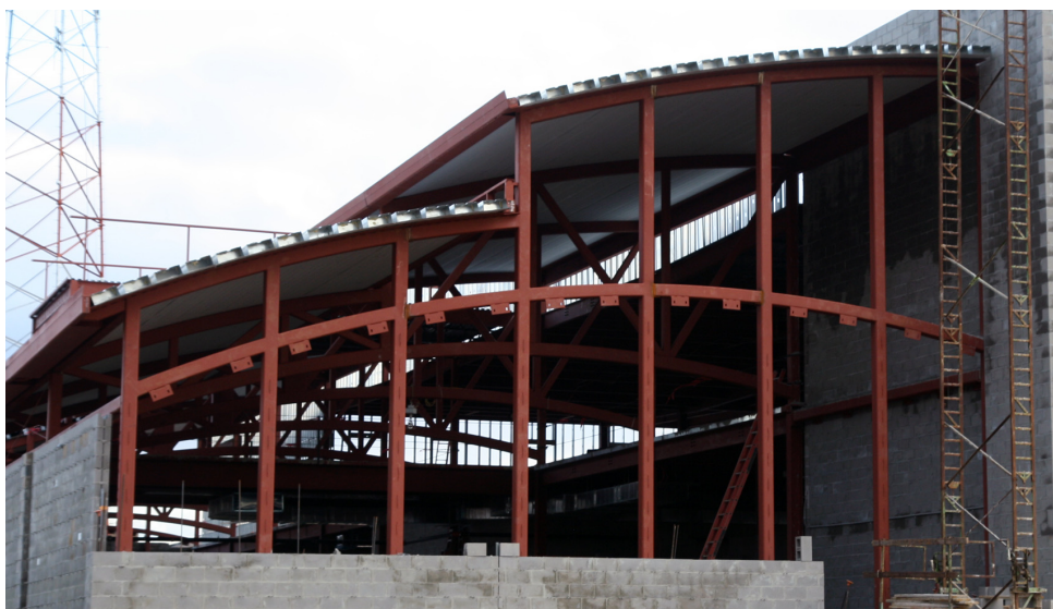
Construction of the county's new 9-1-1 Communications Center is well under way.
